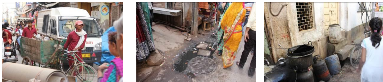
Figure 4.5 Waste collection, water logging on main road and uncovered drains
